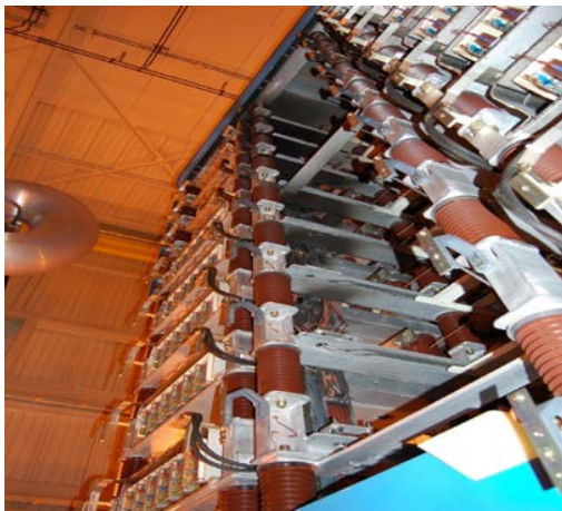
Figure 3.4. Damage caused by flashover due to a water leak in VG32 at Henday on December 04, 2011.
