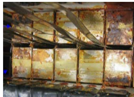
(b) Delaminated core parts.
