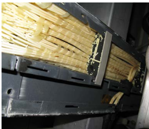
Figure 3.10(a). Severely deteriorated LG insulation jackets at Henday.
