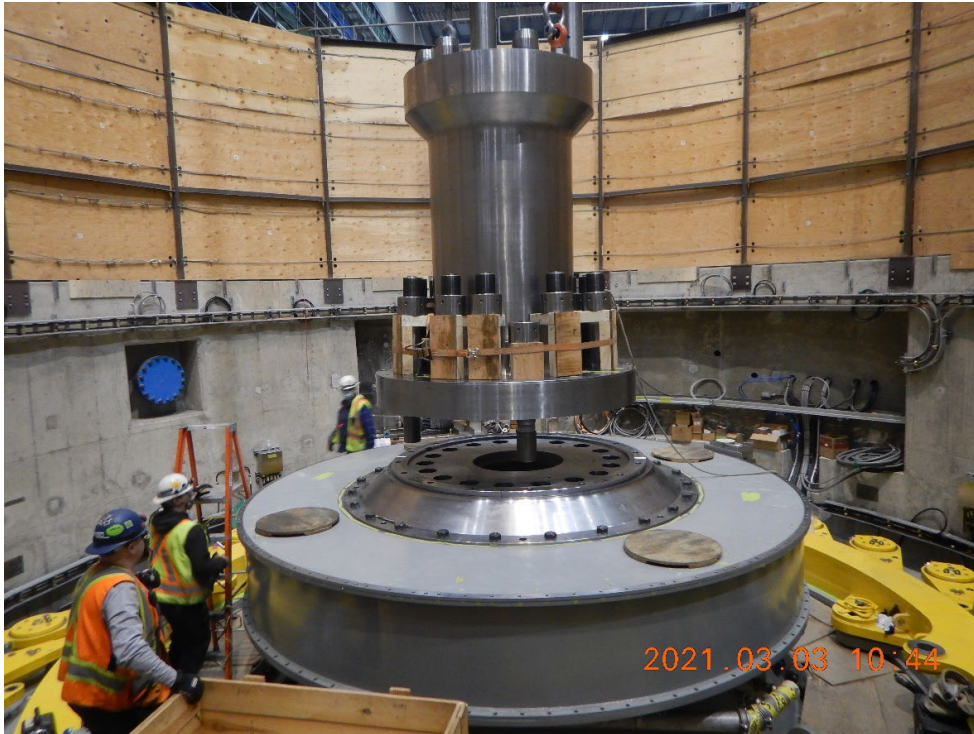
Photo #3: Unit 4 Generator Shaft installation (March 2021)
