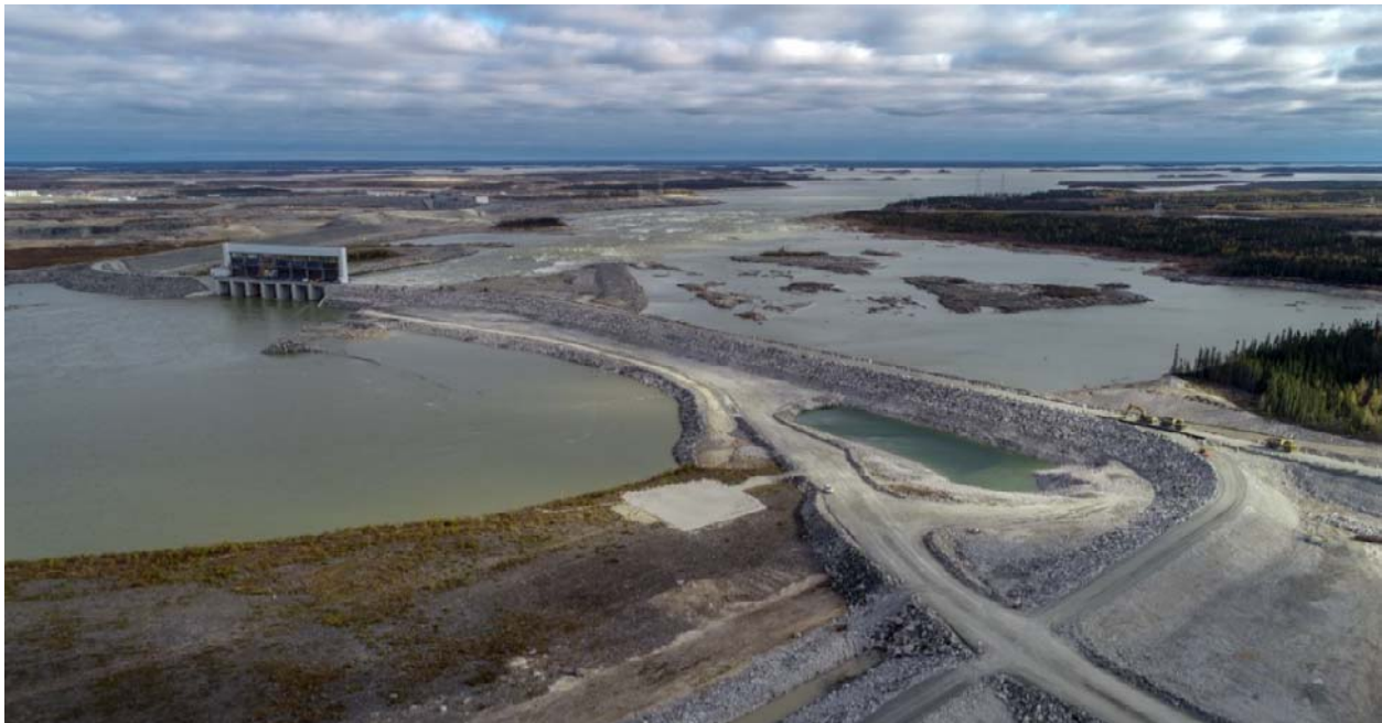
Photo 6: South Dam – September 2019
