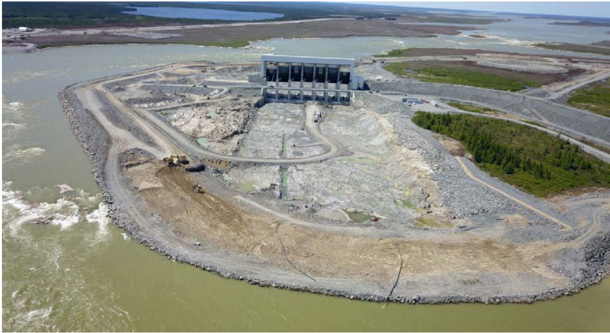
Photo #7: Spillway – June 24, 2018
