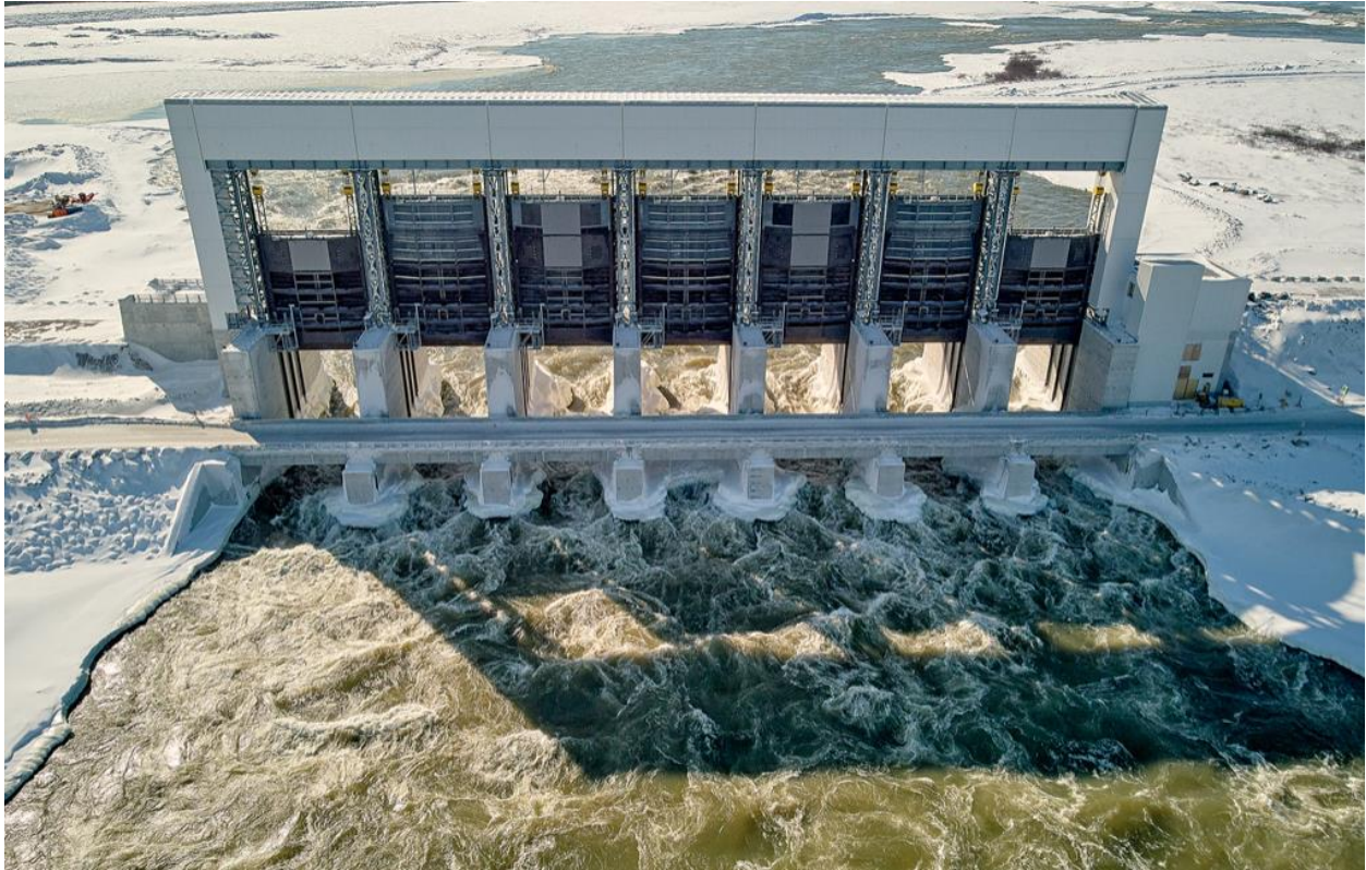
Photo 5: Keeyask Spillway – March 2019
