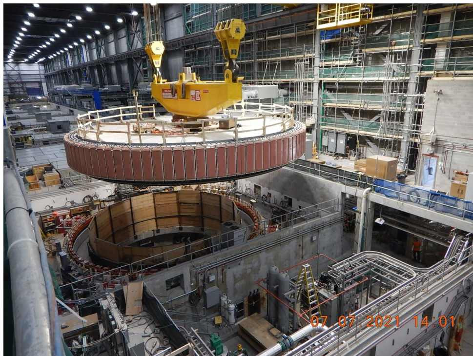
Photo #2: Unit 7 Rotor installation
