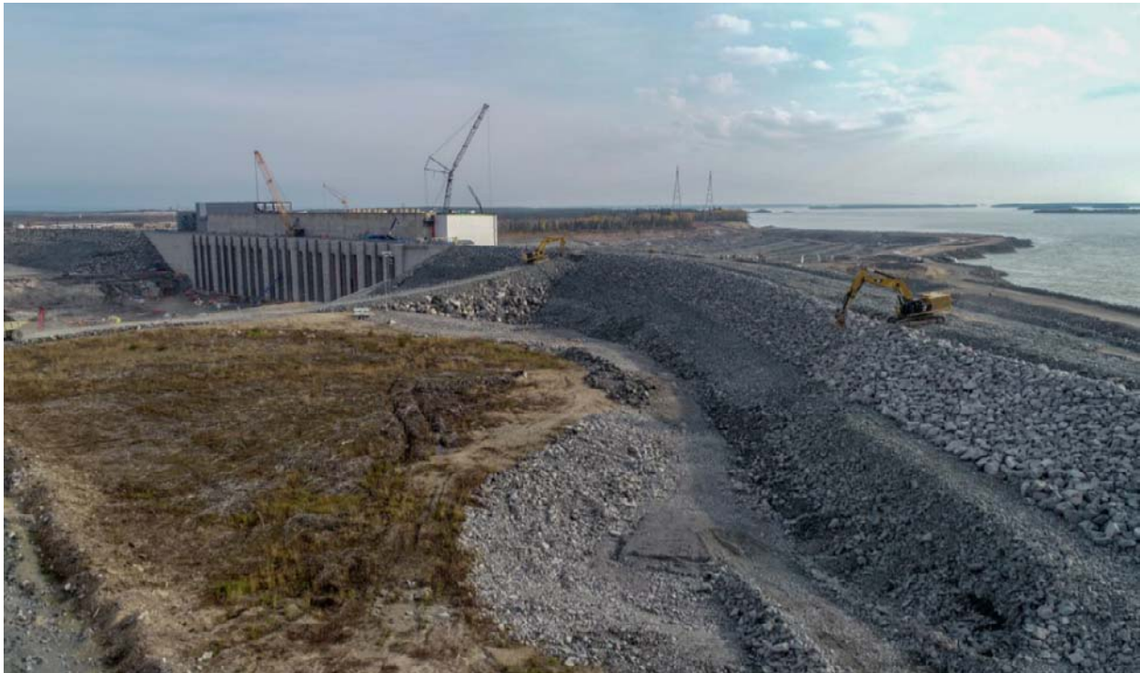
Photo 5: Central Dam Construction – September 2019
