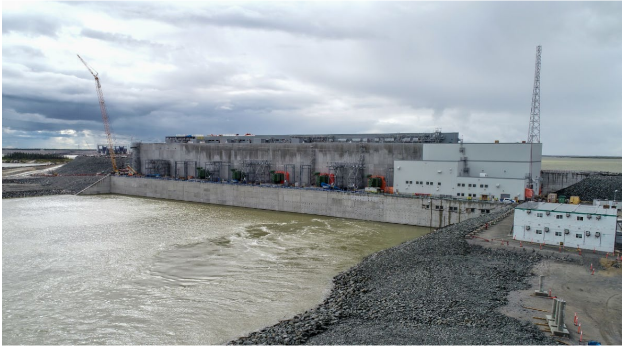
Photo #7: Water Passing Through Unit 1 for the First Time – September 2020
