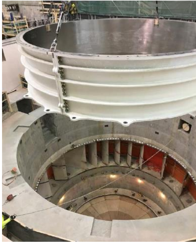
Photo 1: Discharge Ring Installed in Unit 1 Turbine Pit – March 2019
