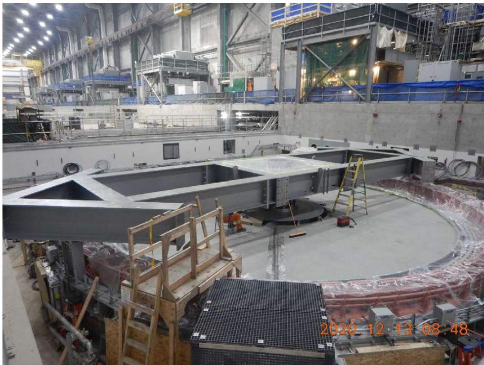
Photo #4: Unit 5 Upper Bracket Installation – December 2020
