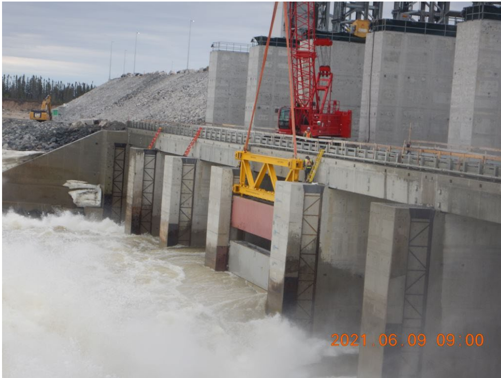
Photo #1: Spillway Water Passage 4 Downstream stoplog removal
