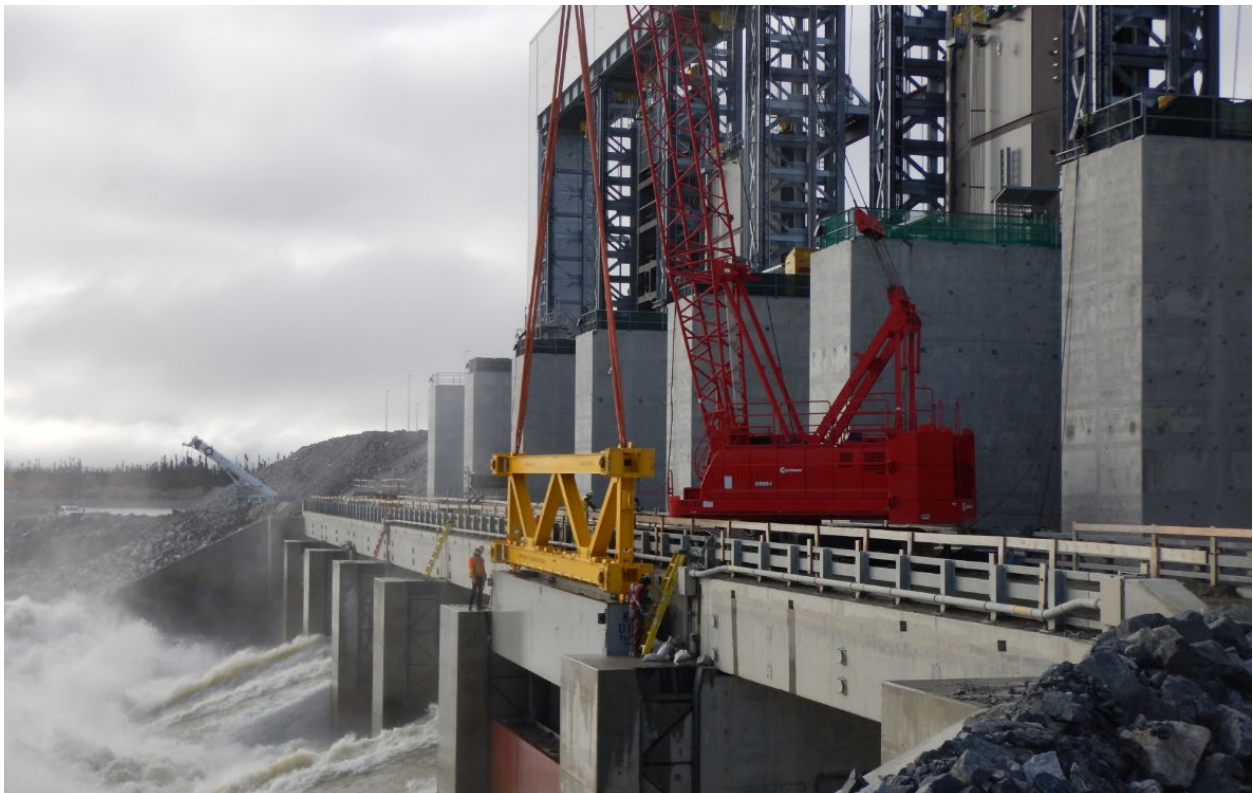
Photo #6: Spillway – September 2020
