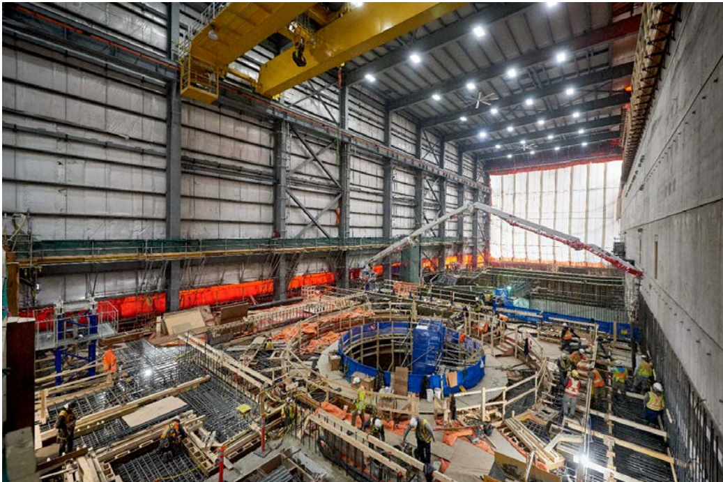
Photo #4: Powerhouse Interior, Embedded Parts for Units 1-3 Installed – November 5, 2018
