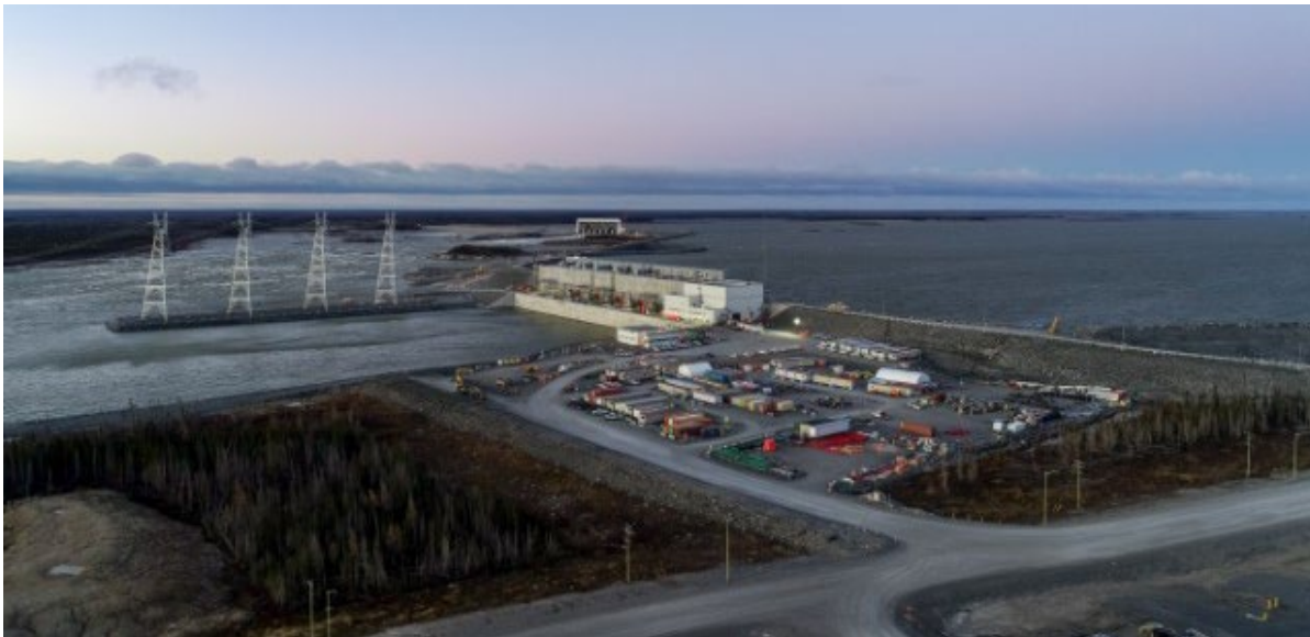
Photo #2: Aerial view of Powerhouse, towers and Spillway – October 2020
