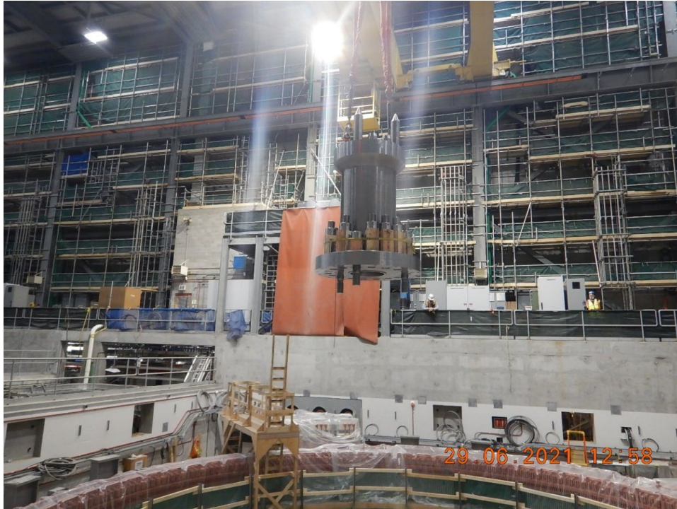
Photo #1: Unit 7 Generator Shaft installation
