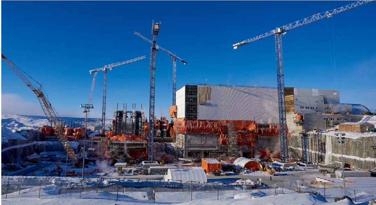
Photo #1: Powerhouse Construction with Units 1 to 3 Enclosed – January 25, 2018
