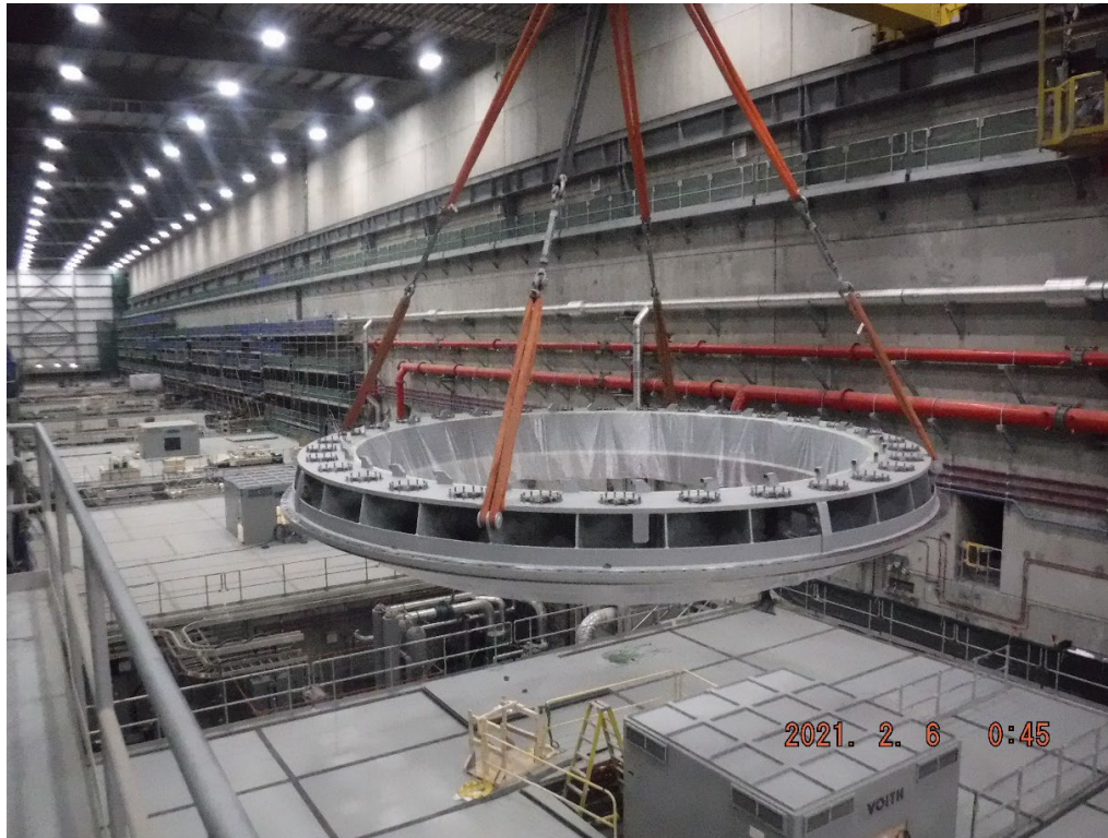
Photo #5: Unit 4 Outer Head Cover Installation (February 2021)
