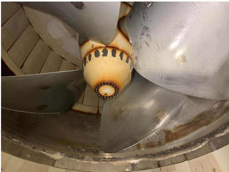
Photo #4: Unit 1 Turbine Runner Inspection Following Online Testing
