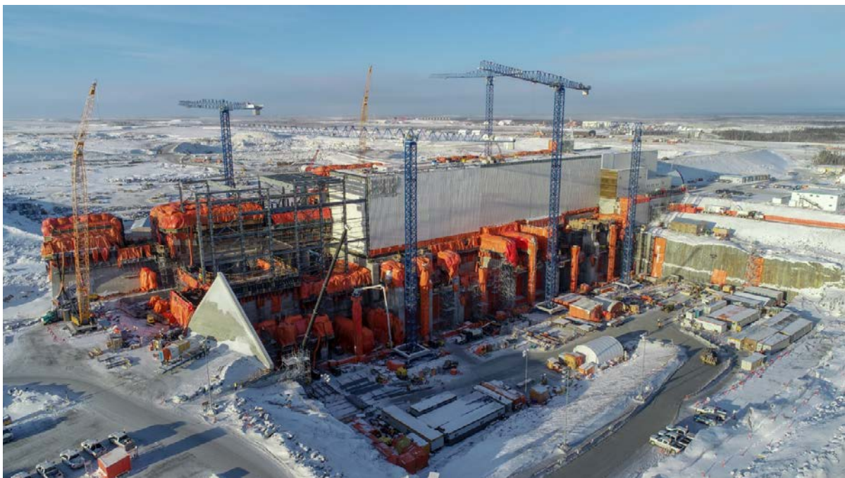
Photo #2: Powerhouse Construction with Units 4 and 5 Now Enclosed – December 9, 2018
