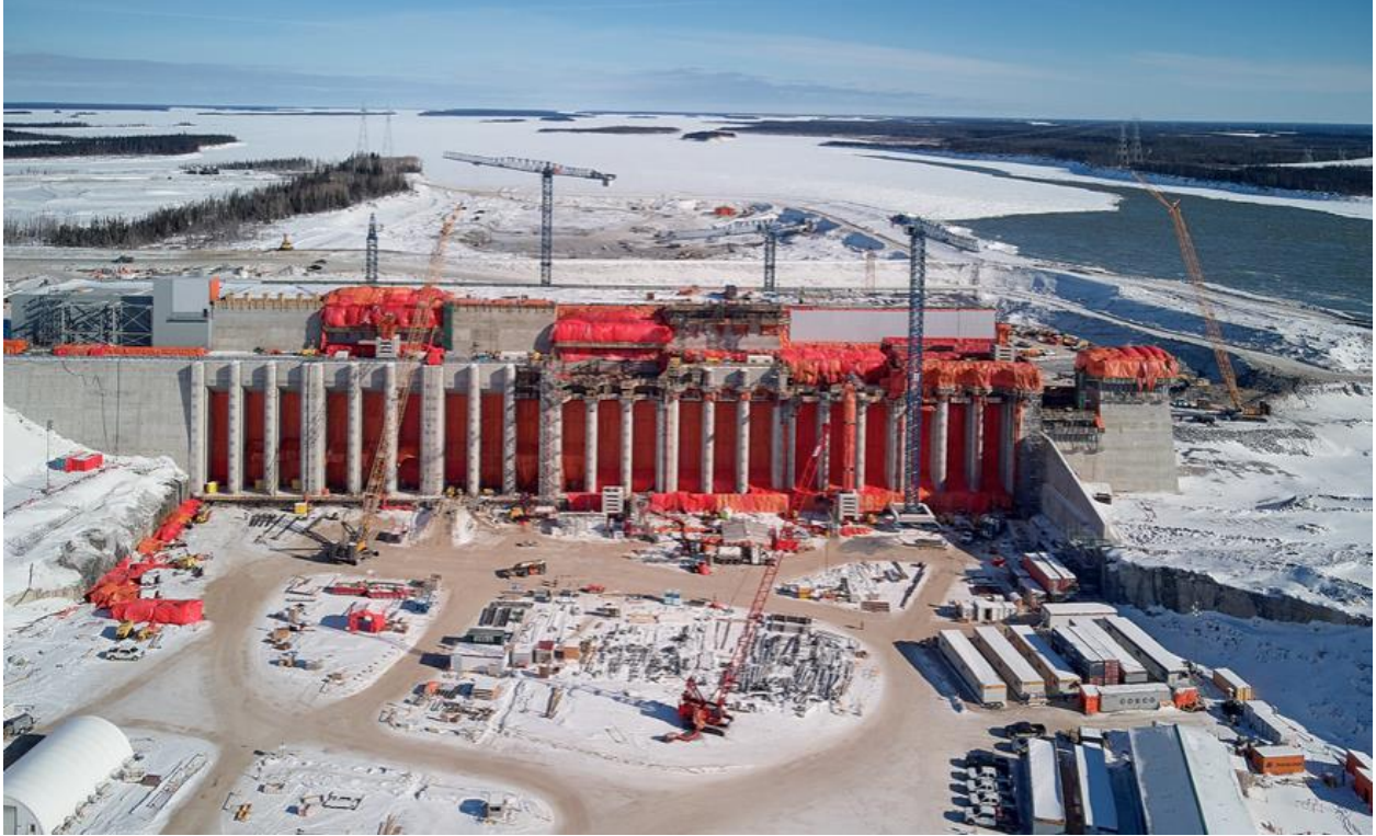
Photo 3: Intake Construction - March 2019
