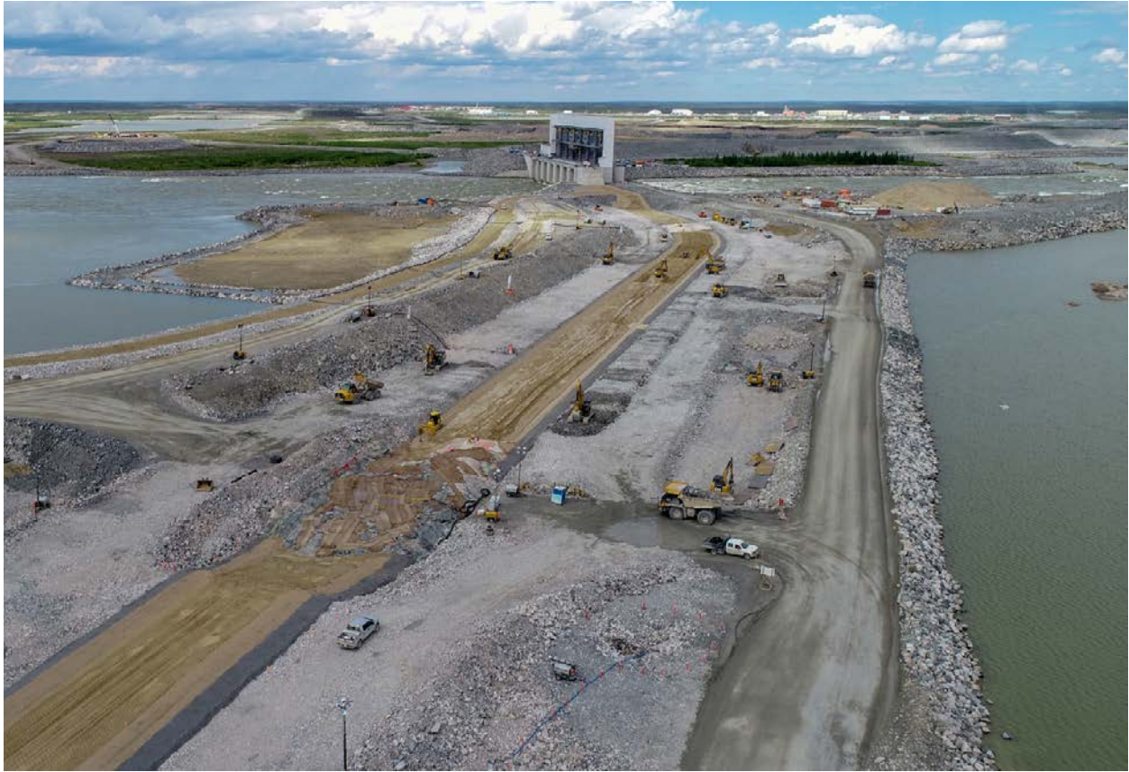
Photo 5: South Dam – June 2019
