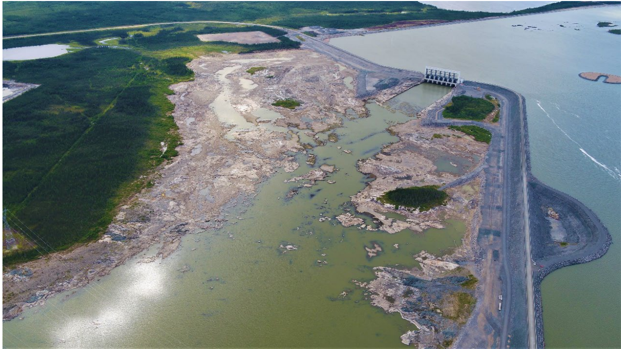
Photo #3: First Spillway Closure Since River Diversion in August 2018
