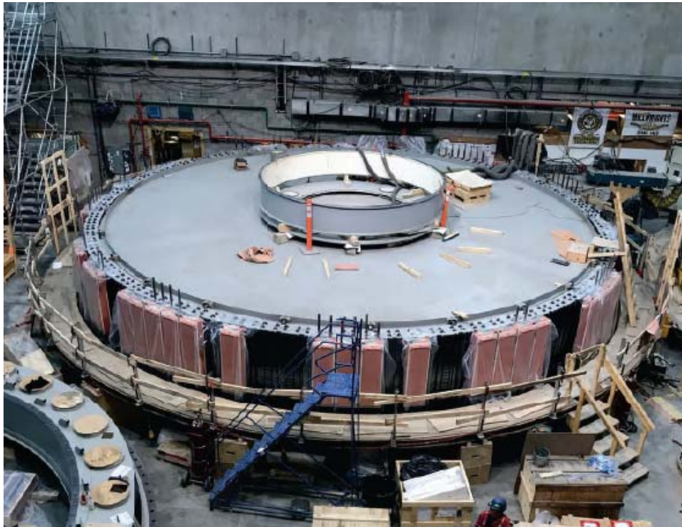
Photo 4: Unit 1 Outer Headcover being lowered into place – September 2019
