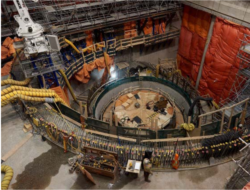
Photo #4: Powerhouse Interior, Embedded Parts for Units 1-3 Installed – November 5, 2018
