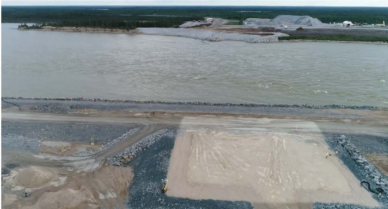
Photo #11: South Dam – early July 2018
