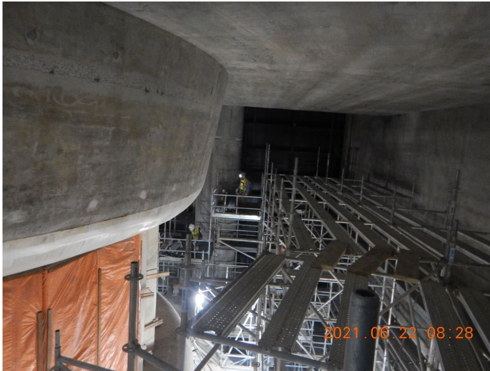
Photo #3: Dismantling Scaffolding in the Upstream of Unit 7 Scroll case
