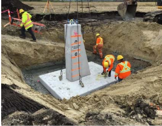
Foundation Installation
