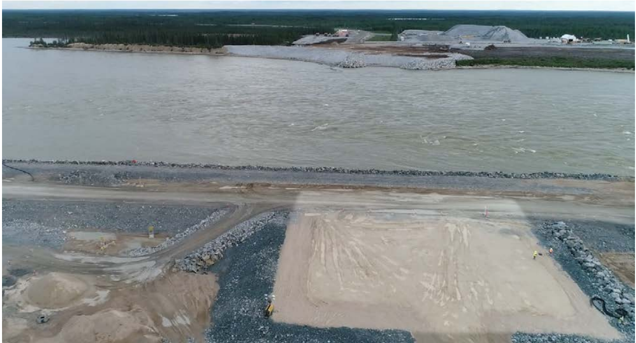
Photo #11: South Dam – early July 2018
