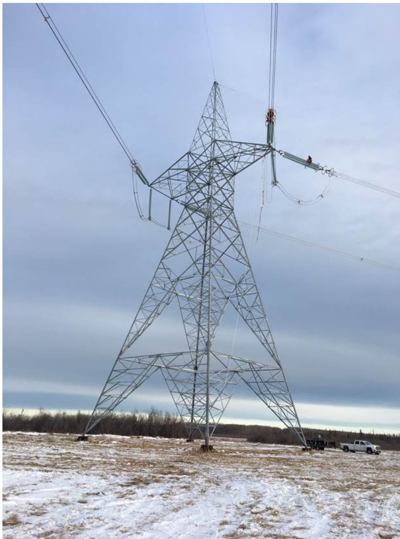
Bipole III transmission tower - N4 –addition of corona ring stiffeners
