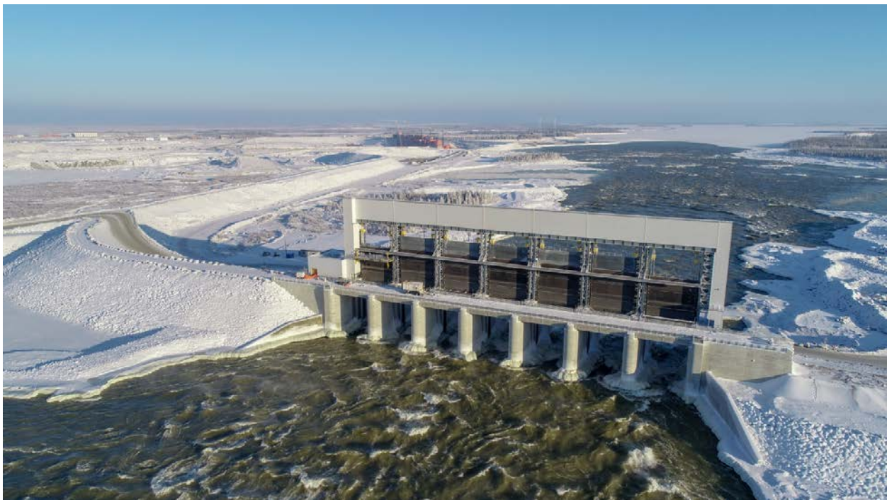
Photo #8: Spillway – December 12, 2018
