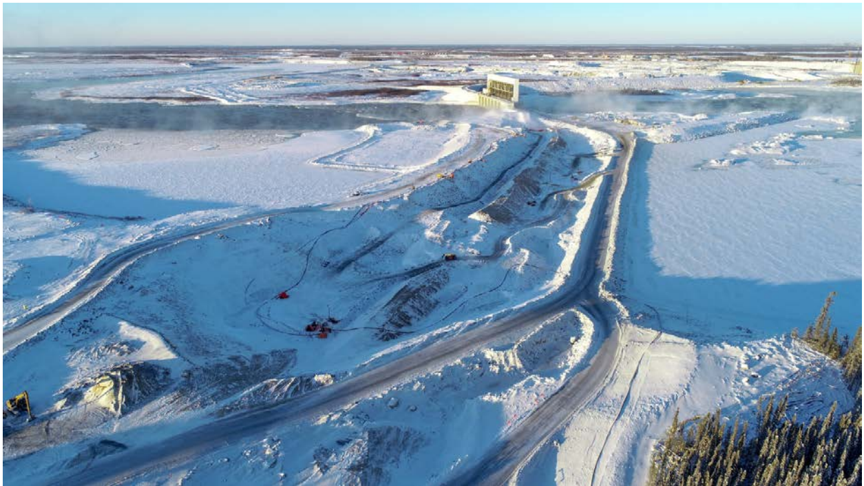
Photo #12: South Dam – December 5, 2018
