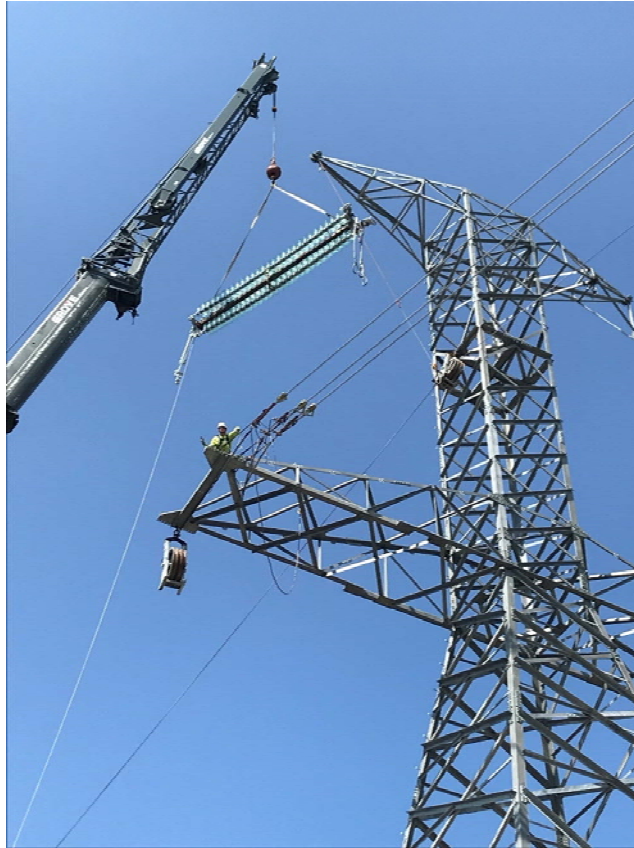
Photo 4: Segment 3 – Dolly Installation
