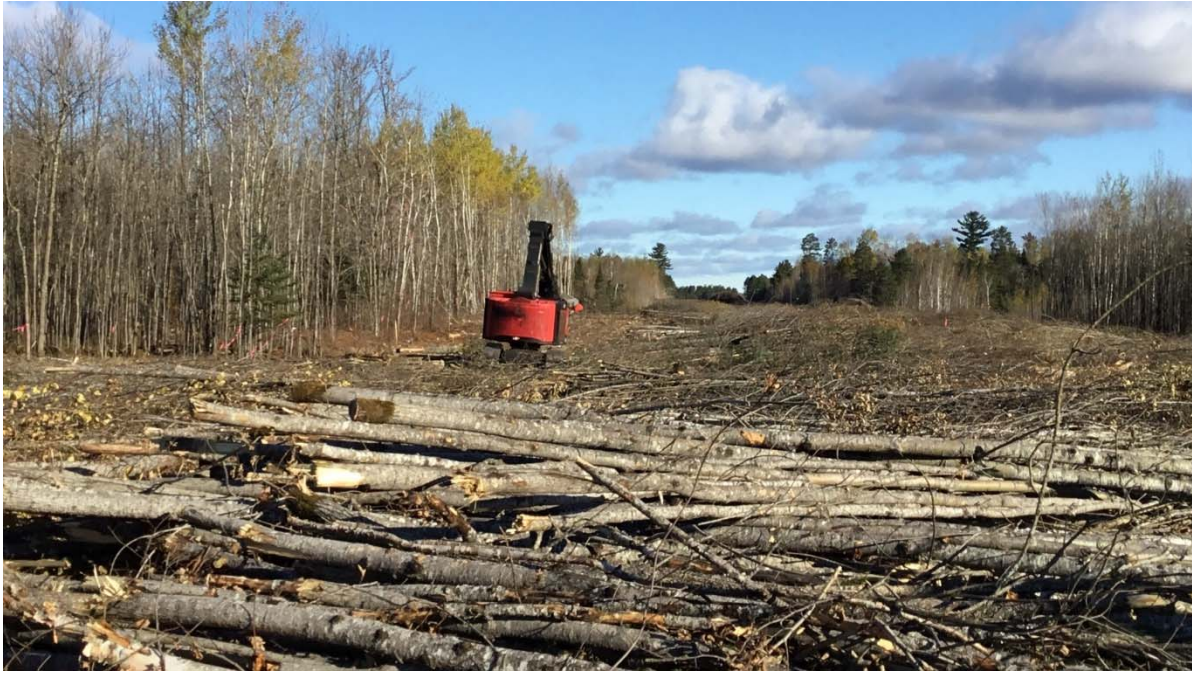
Photo 5: Segment 4 – ROW Clearing
