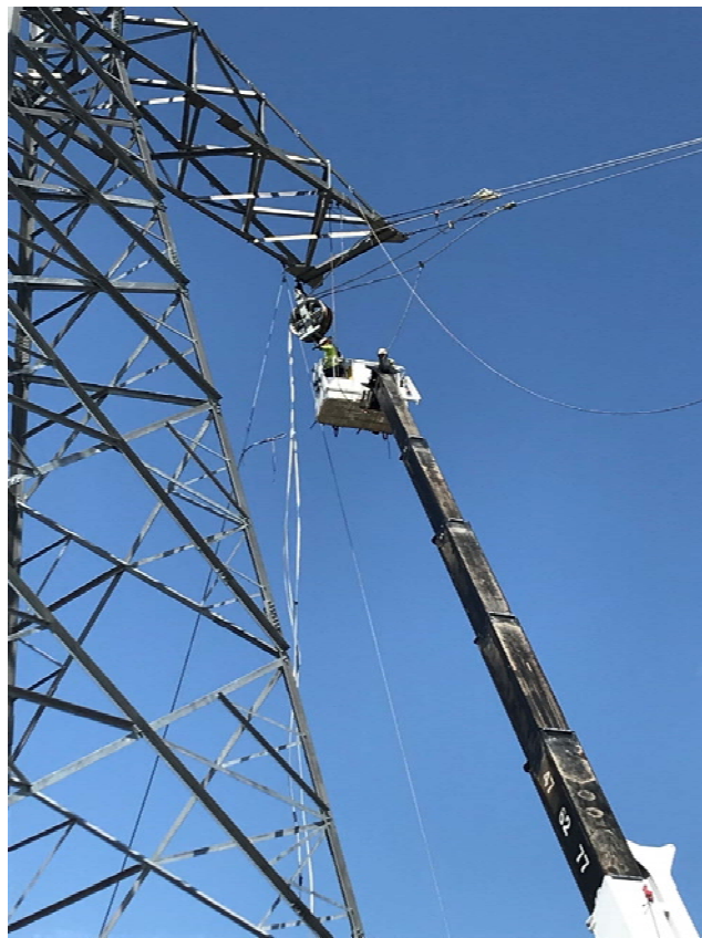
Photo 4: Segment 3 – Dolly Installation
