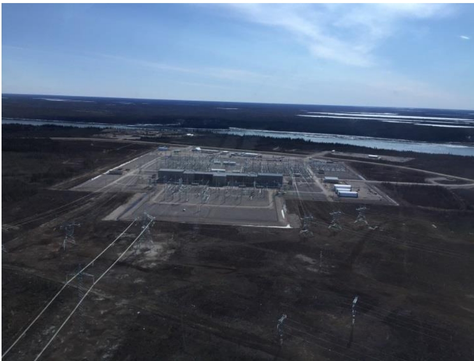
Photo 6: N1 – Keewatinohk Converter Station
