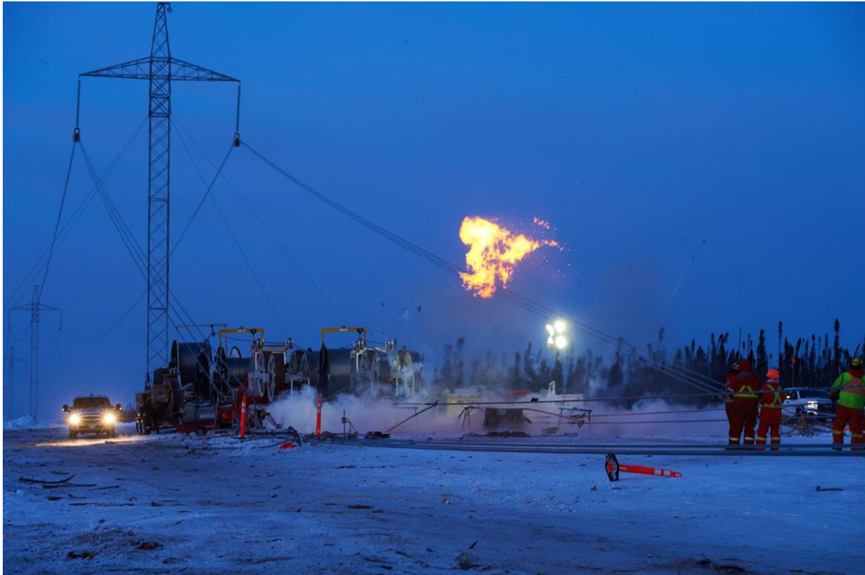
Photo 3: Bipole III N1 Stringing Operations – Implosive Sleeve Detonation
