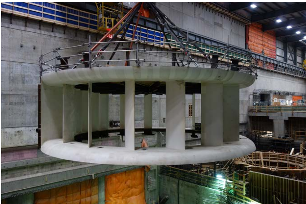
Photo #2: Installation of the Unit 2 Stay Ring (Turbine and Generator embedded component) – September 18, 2018
