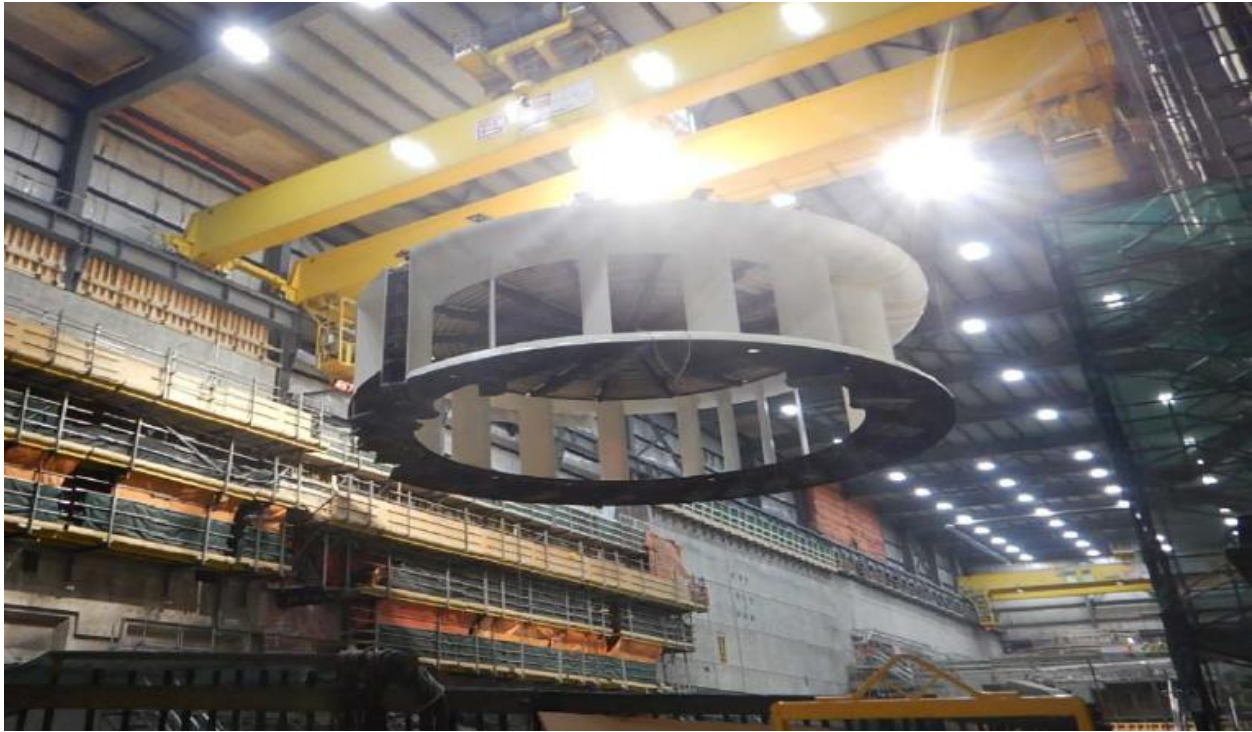
Photo #5 – Lowering Unit 3 Stay Ring into Place – June 11, 2018
