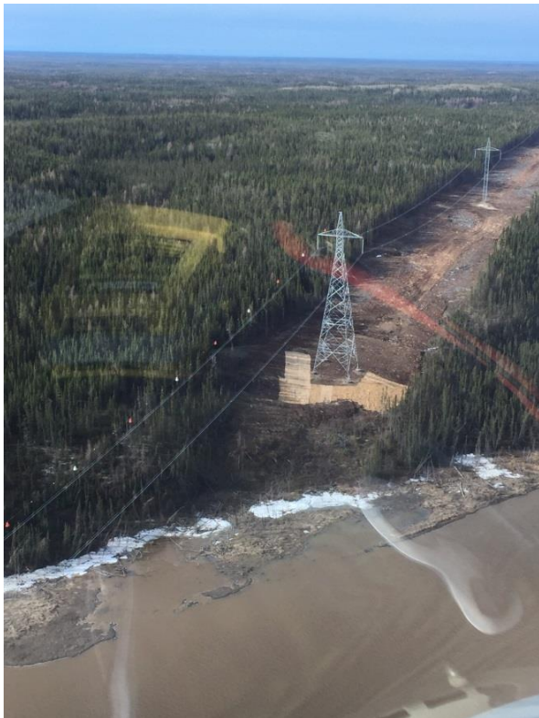
Photo: N1 – Environmental Inspection STR 517
