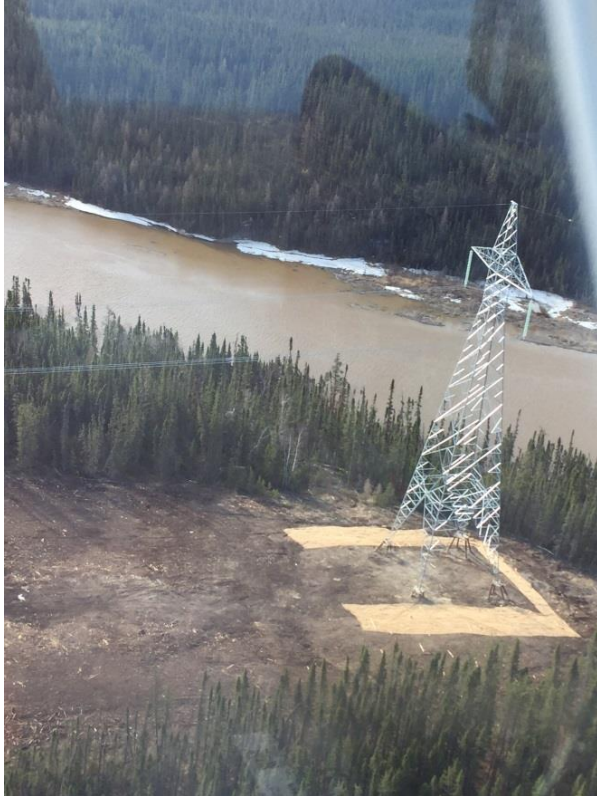
Photo 3: N1 – Environmental Inspection STR 516
