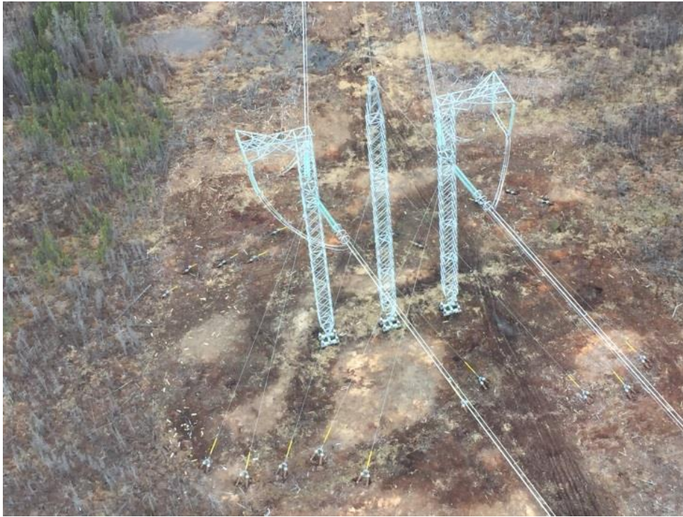
Photo 5: N1 – C530 Guyed Tower
