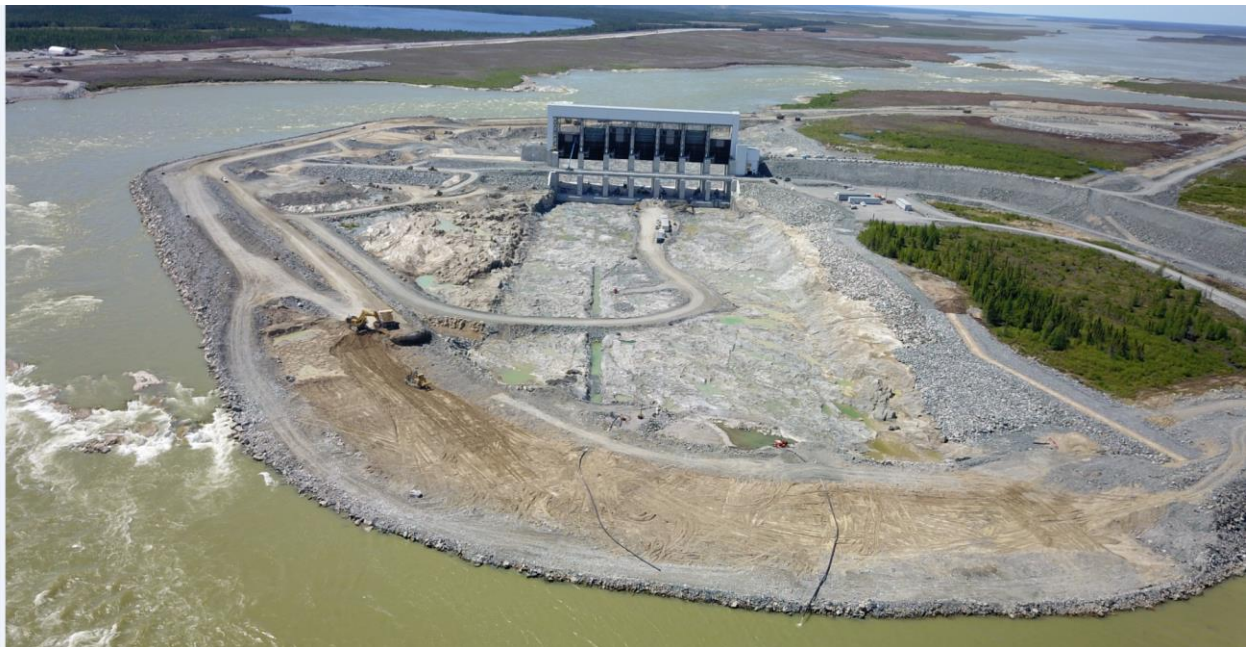
Photo #2: Aerial View of the Spillway and Spillway Cofferdam Removal “in the dry” – June 18, 2018
