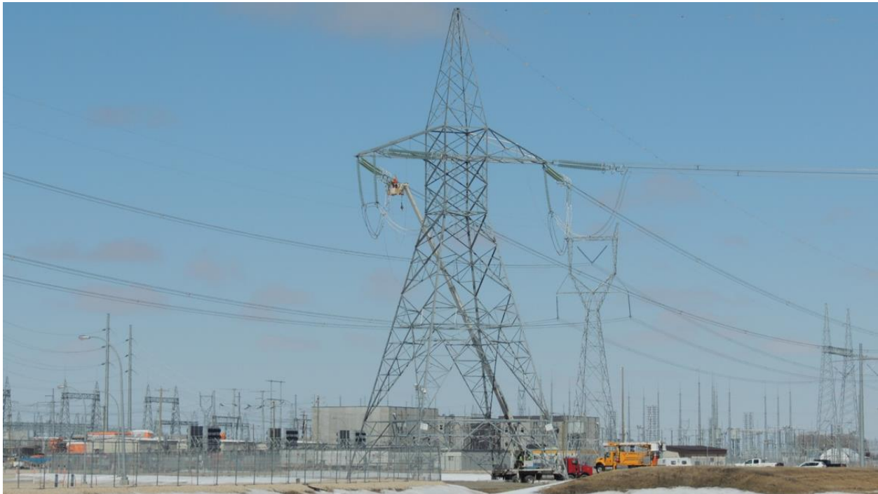
Photo 4: S2 Tower #7338 RCS Final Jumper Installations March 31, 2018
