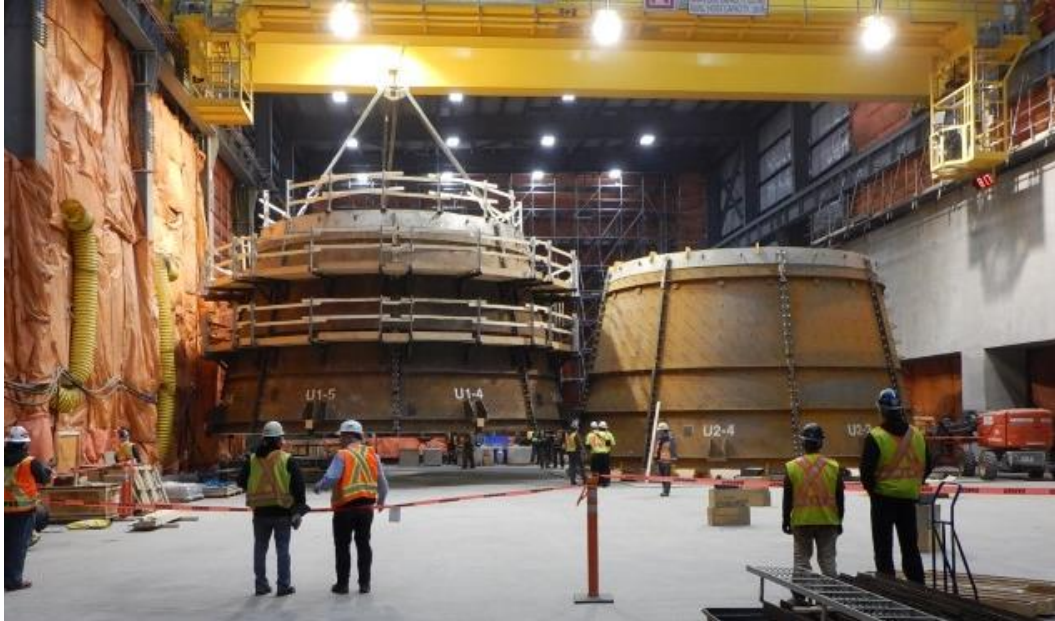
Photo #2: Unit 1 Draft Tube Liner Installation by the Turbine and Generator Contractor – January 21, 2018
