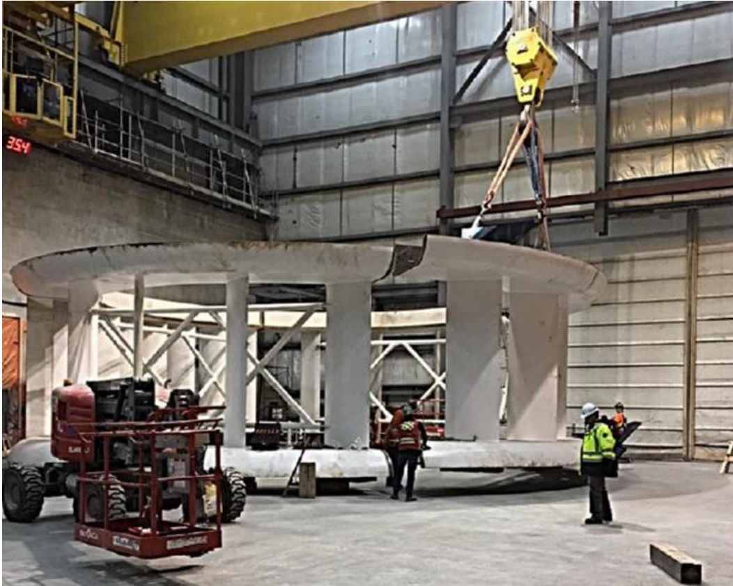
Photo #5: Stay Ring Assembly by the Turbine and Generator Contractor – March 29, 2018
