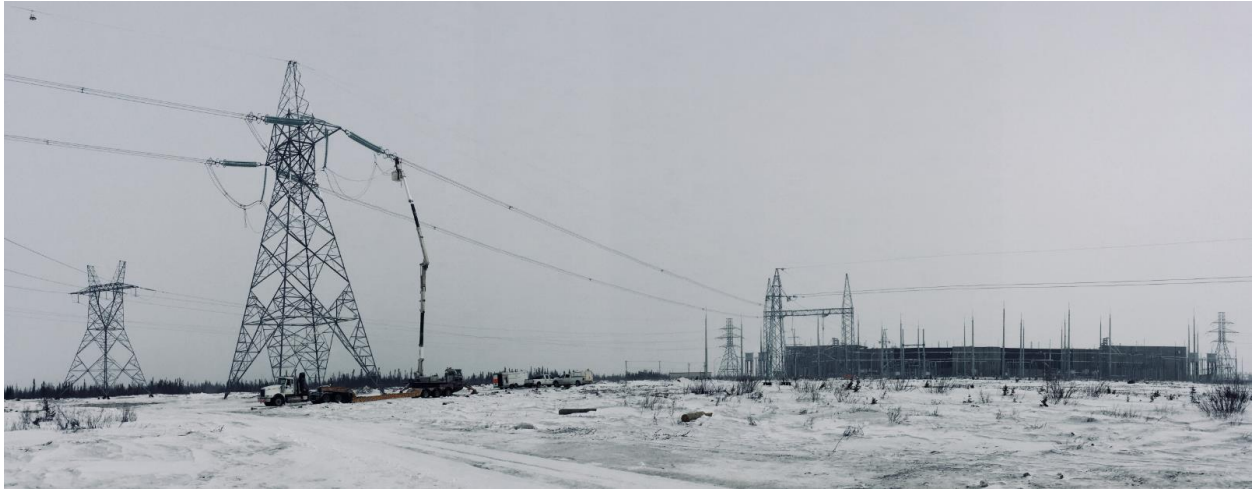
Photo 1: Final Jumper connections, N1 Tower #1 at Kewatinohk Converter Station
