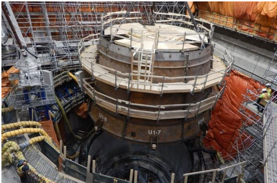
Photo #2: Unit 1 Draft Tube Liner Installation by the Turbine and Generator Contractor – January 21, 2018
