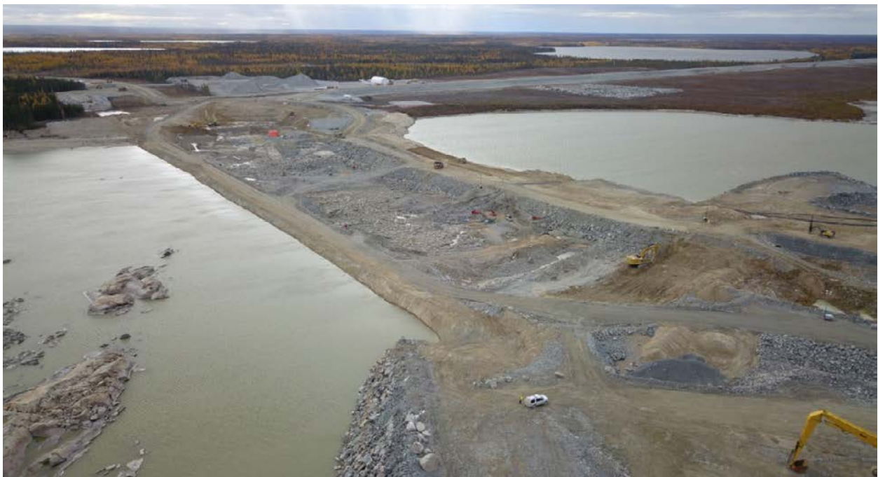
Photo #6: Dewatering and Excavation within the South Dam Cofferdam – September 30, 2018
