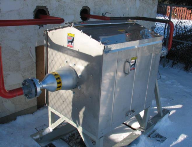
Figure 4.7 – Catalytic pipeline heater
