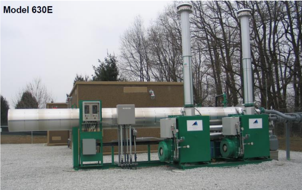
Figure 4.8 – CWT 630E line heater
