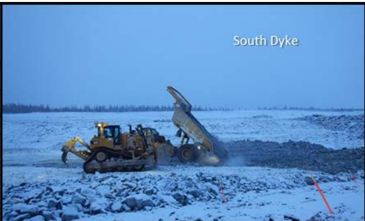
Dozer (05-23) placing Class 6 material that is being hauled in by 773 haul trucks from Quarry Q1. Sta. SD 19+425 to SD 19+405
