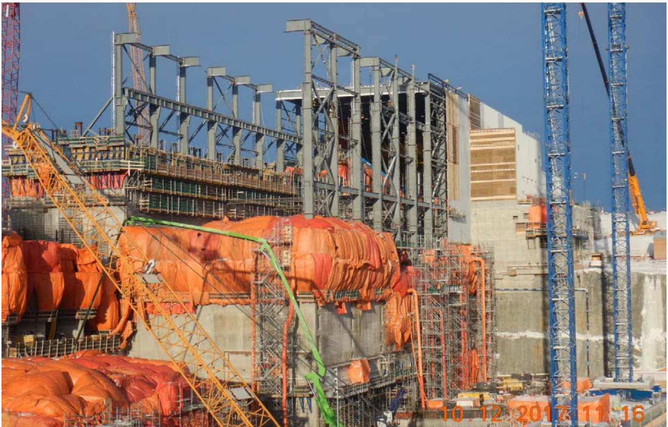
View of structural steel progress on Powerhouse Units 1 to 3
