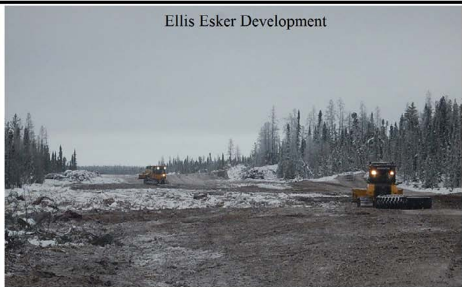
Dozers continued dragging roadway towards to Ellis Esker between Sta. 0+000 to approximately 5+700
