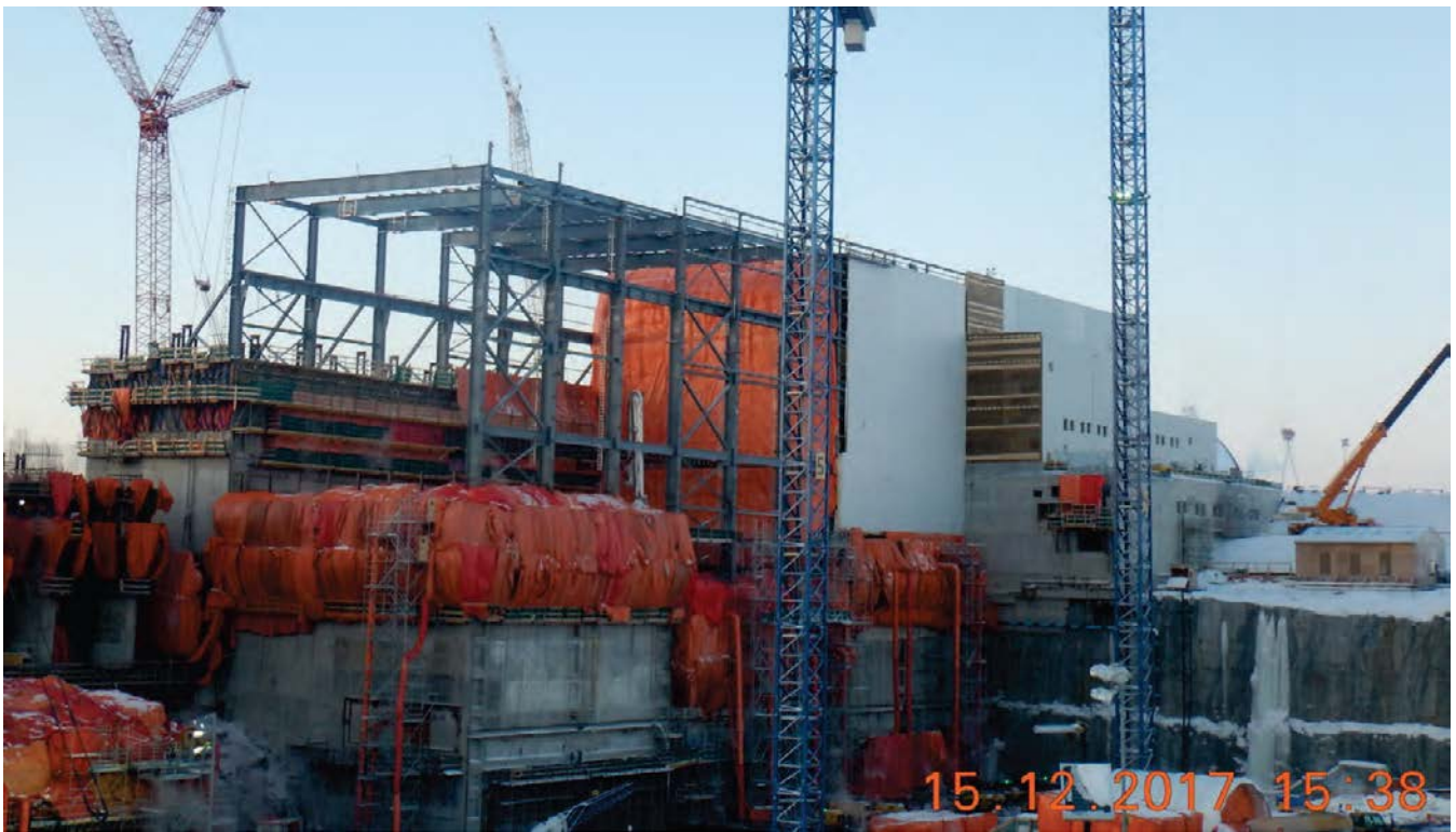
View of the service bay and powerhouse enclosure
