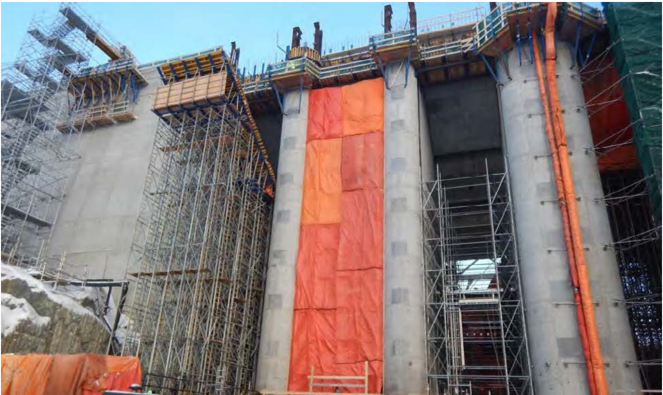
Intake 1 water passage 1 removal of headblock shoring
