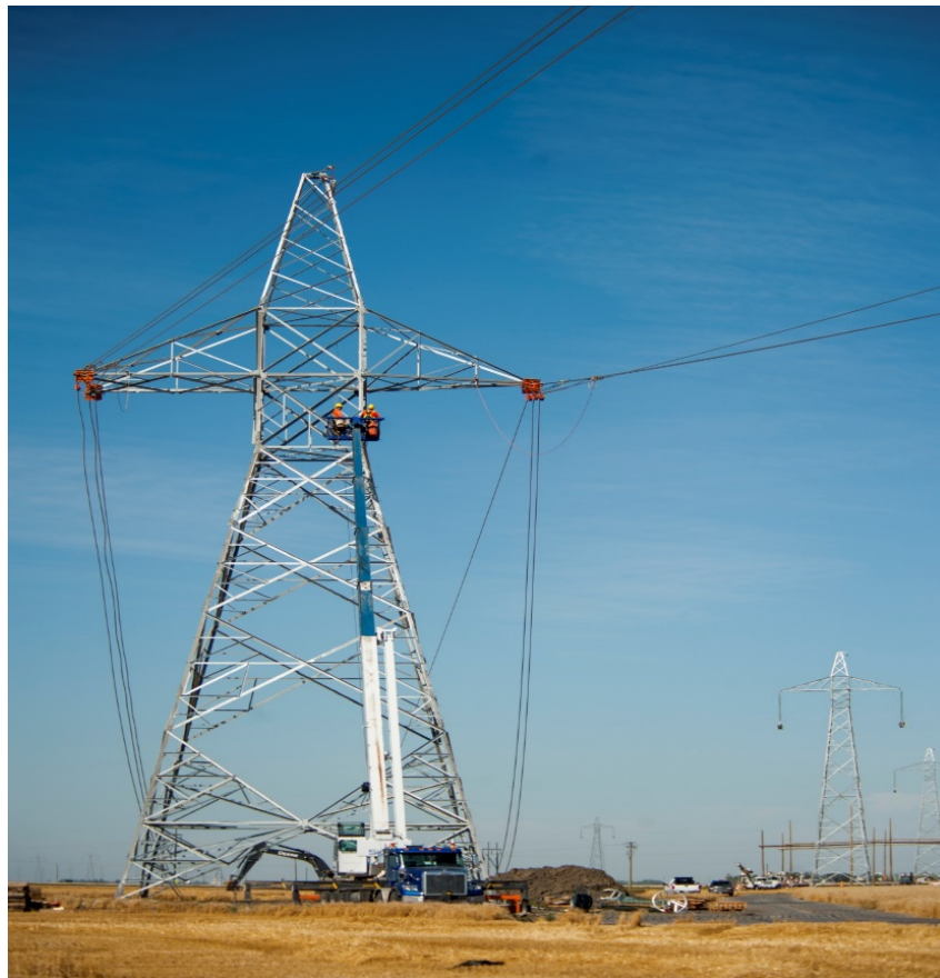
photograph provided by Manitoba Hydro
