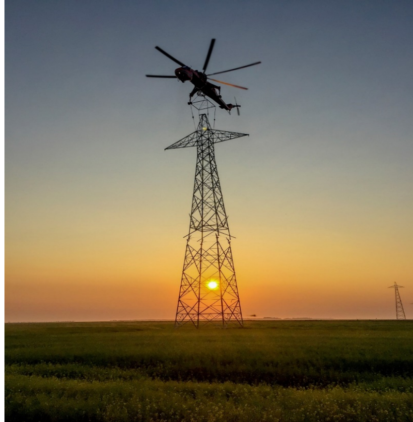
photograph provided by Manitoba Hydro
