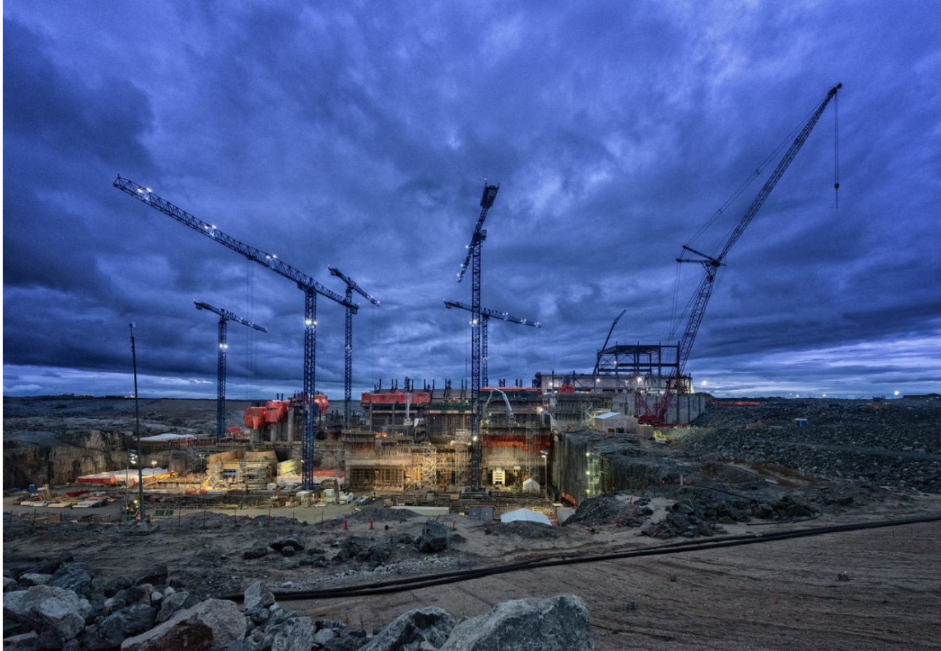
Powerhouse Complex July 2017 photograph provided by Manitoba Hydro
