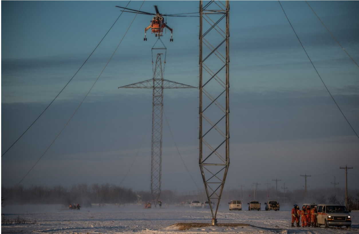
photograph provided by Manitoba Hydro
