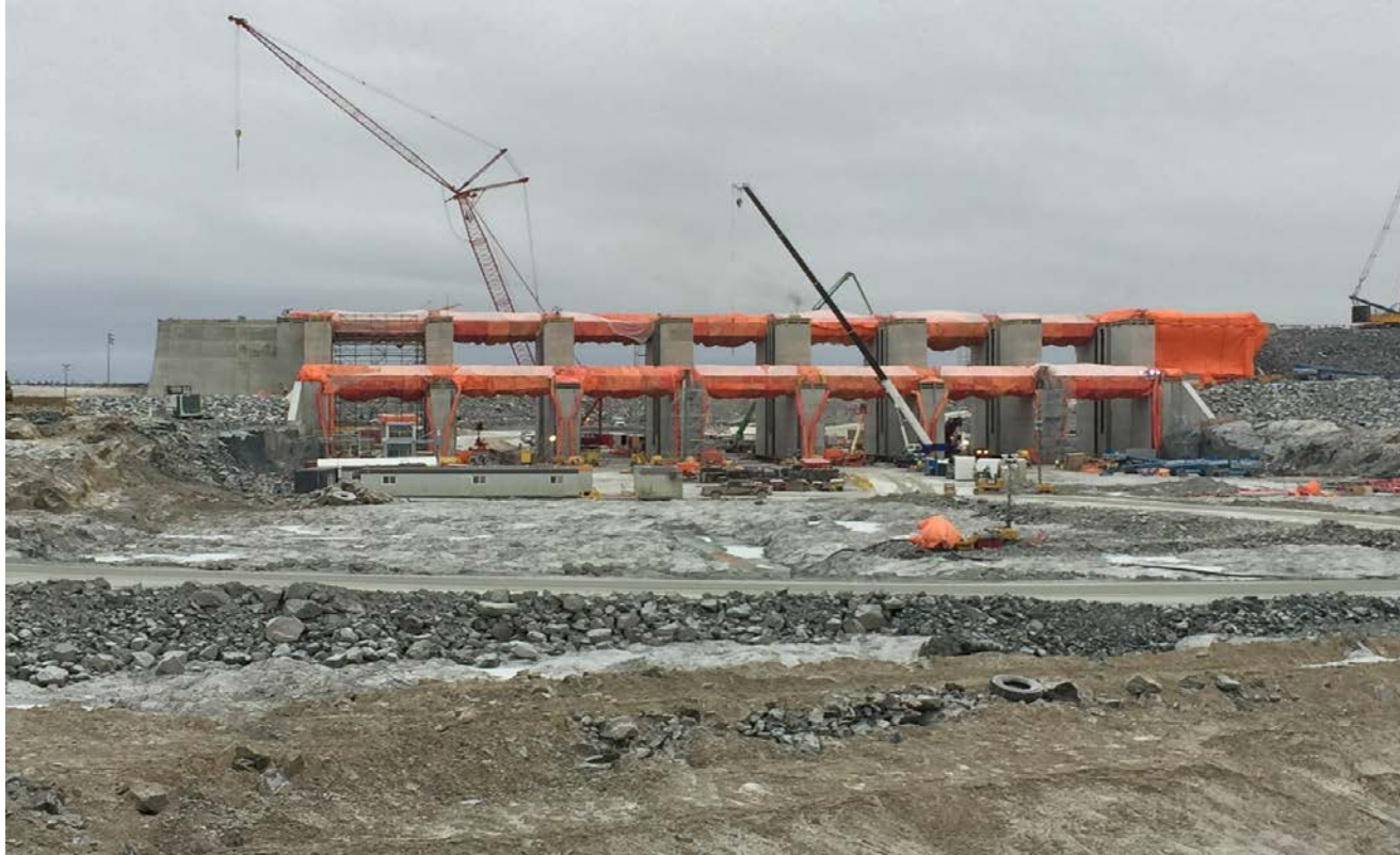
Spillway October 2017 photograph provided by Manitoba Hydro
