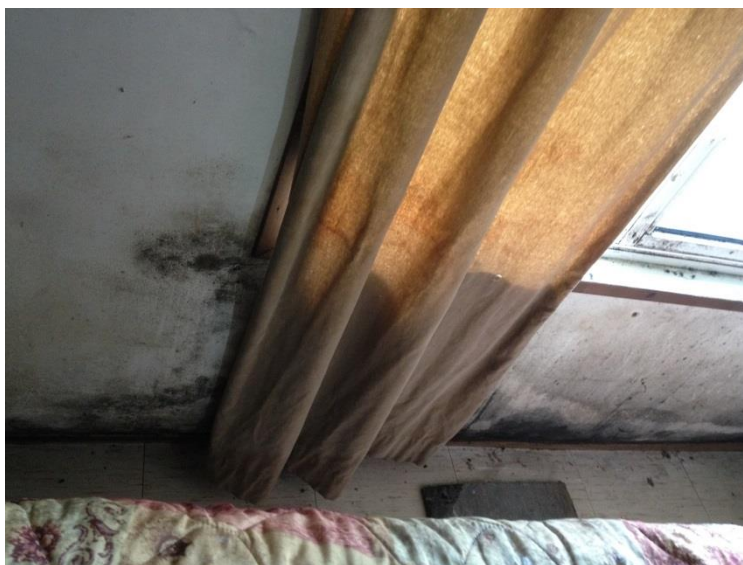
Photo: Mould in a bedroom shared by several children. (Sandy Lake First Nation, Ontario)
