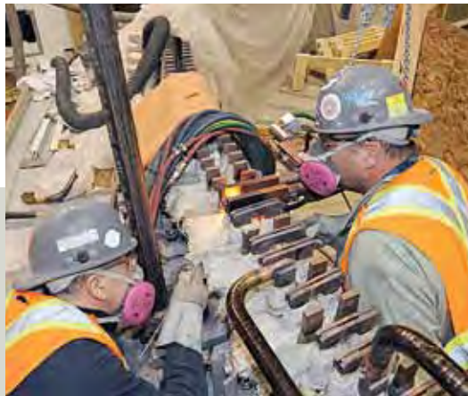
Top: Opening the river. Bottom: Wuskwatim construction.
