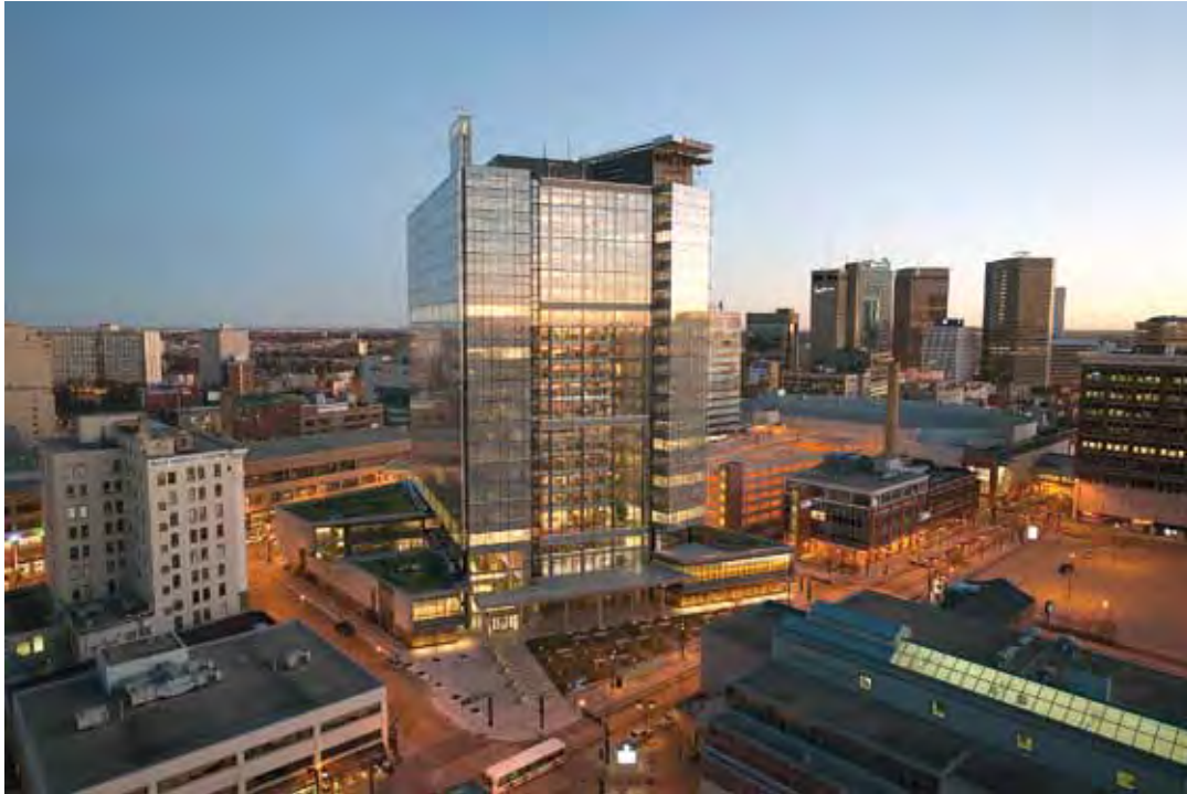
Manitoba Hydro Place
