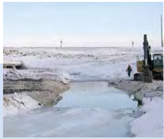
Sturgeon Creek bypass dams and pumps removed with some bank restoration still required. The 16" pipeline now runs under the Sturgeon Creek.
