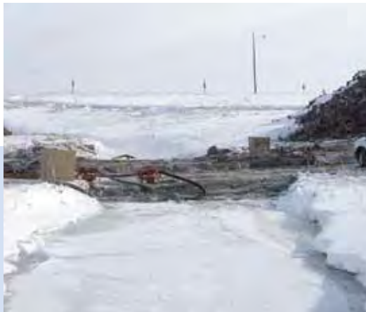
View of the Sturgeon Creek bypass looking downstream.
