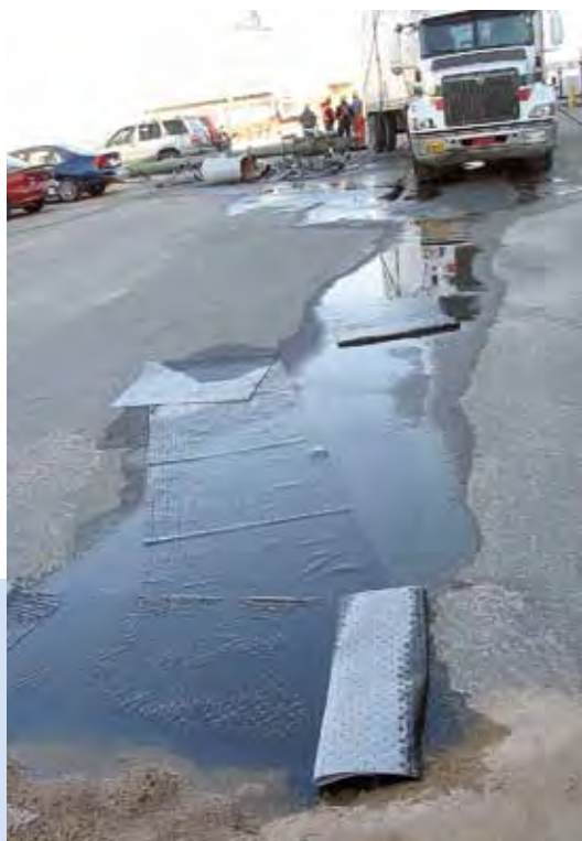
Absorbent pads capture oil on the asphalt surface.
