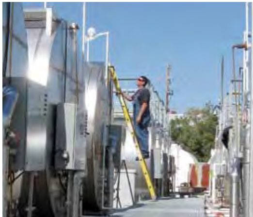
Tanks containing recycled oil at the Waverley Service Centre.
